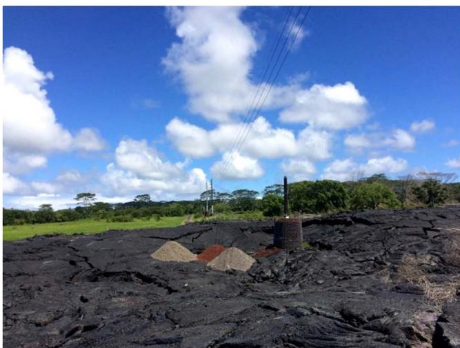
**Fig. 3.** Top left: Photo of active pahoehoe lava flows encircling a utility pole that had been lifted and buffered with cinder blocks as a preventative action (Photo credit: Hawaiian Electric Light Company). Top right and bottom: Photos of utility pole roughly one year after lava had passed through (Photo credit: Nicole Lautze).
